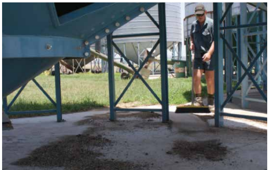
Figure 7: Concrete slab under silo makes cleaning up spilled grain much easier.
