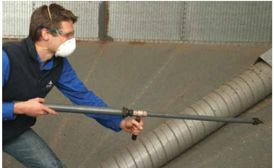
Figure 6: Clean silos, including the silo wall, with air and/or water to provide a residue-free surface to apply structural treatments.
