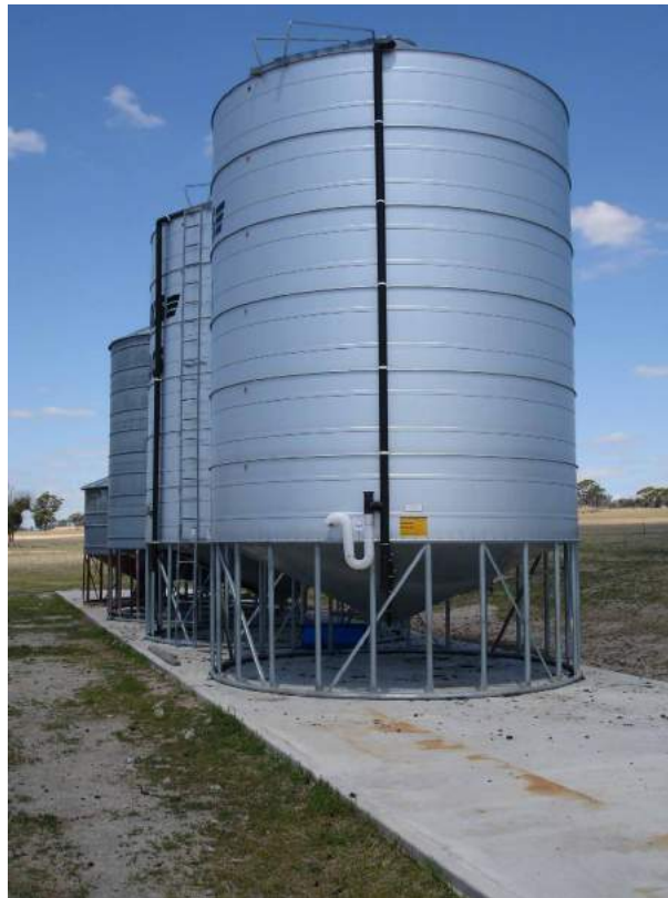
Figure 2: On-farm grain storage silos in one of the first trials in Western Australia assessing seed quality in on-farm storage systems.
