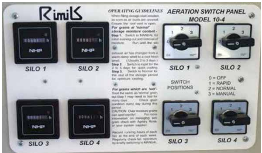
Figure 12: Automatic aeration controllers are the most effective way to cool grain and are designed to manage many storages, from one central control unit.
